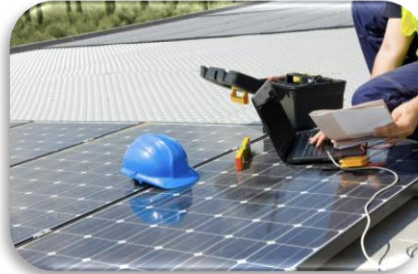
Electrical inspection service
