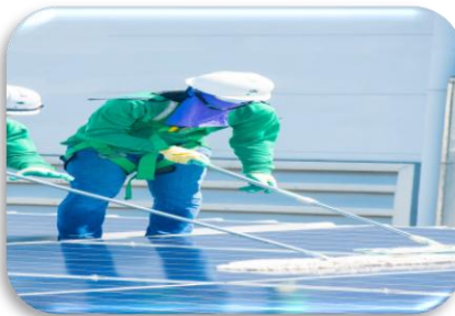
Cleaning and coating service
