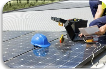
Electrical inspection service
