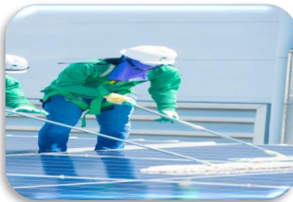
Cleaning and coating service
